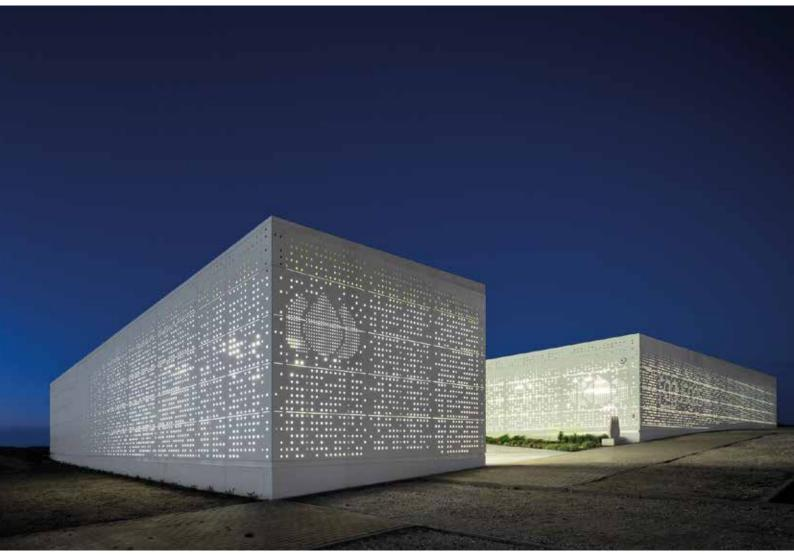
**SwissPearl**<sup>®</sup> is a high-tech fiber cement composite panel, manufactured in Switzerland and marketed all over the world. Certified according to ISO 9001 and endowed with remarkable resistance to the elements, **SwissPearl**<sup>®</sup> panels have a life expectancy of more than 50 years.
